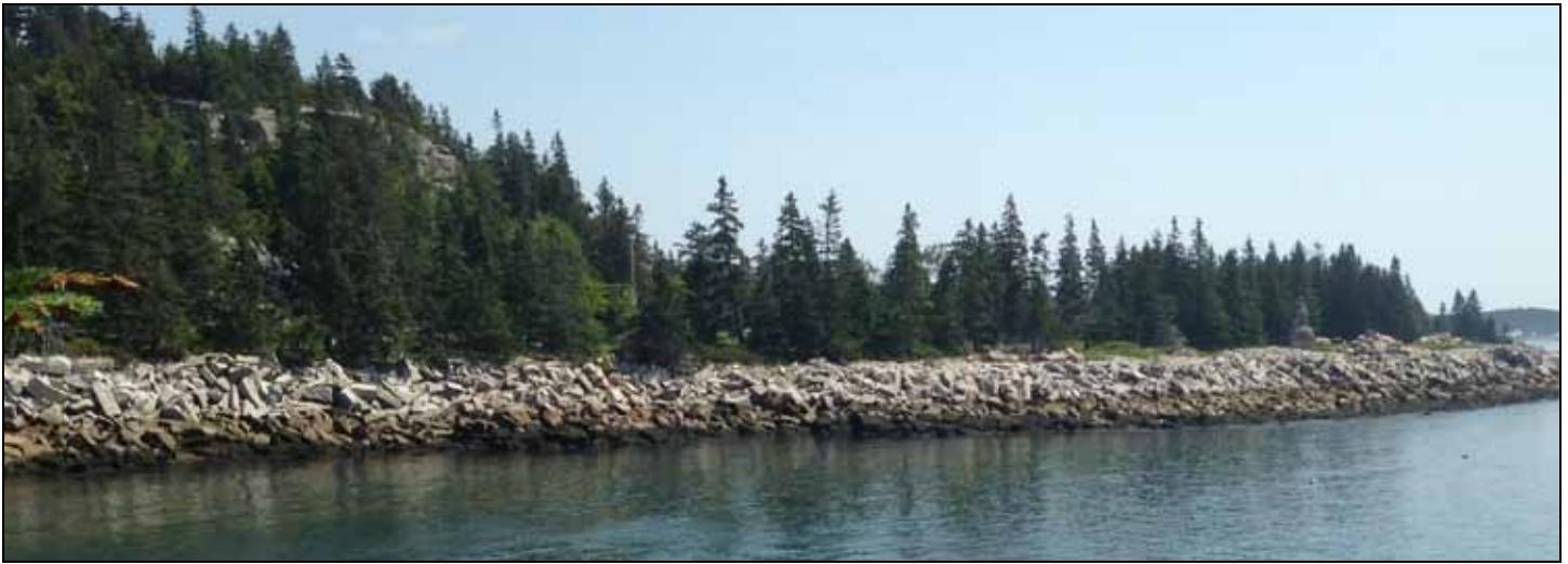
Fig. 30: Discarded quarry stones piled up along the southeastern shore in Gaston Cove.
